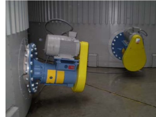
Plenty Fixed Angle Belt Drive Mixers installed on a heated tank
